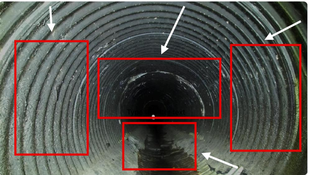
White mineral deposits and efflorescence along the right-hand wall indicate moisture ingress and possible deterioration at the joints (0.20)
